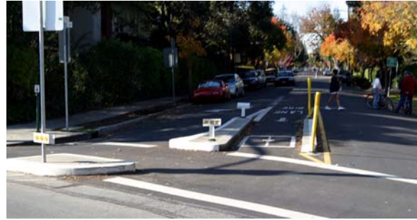
Example traffic diversion at intersection
