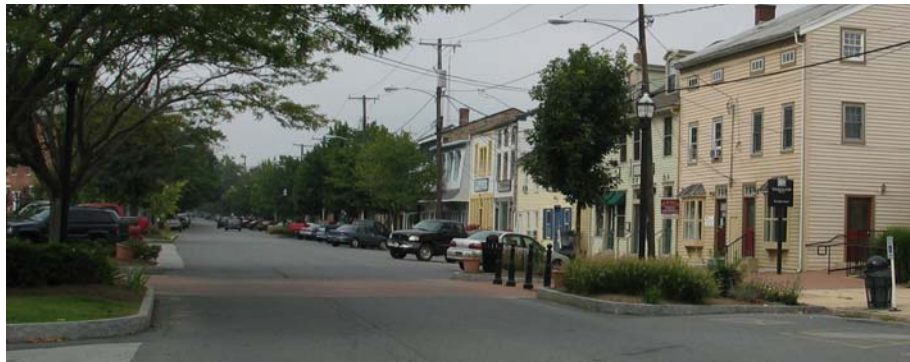
Existing neckdown on Clinton Street
